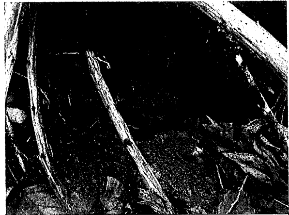
Photo 6 – silty sand and gravel soil exposed on slope
