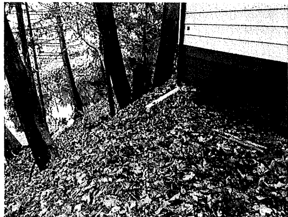
Photo 3 – Ground settlement at southeastern corner of #115
