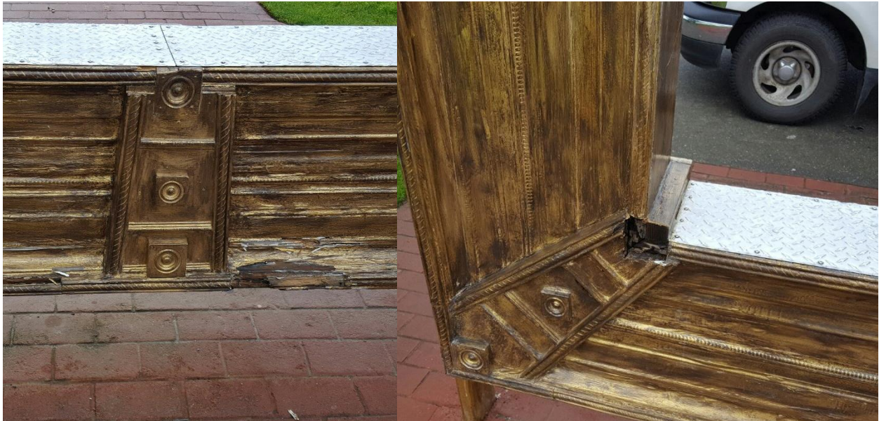
Dry rot and deterioration returned in 2017 unabated due to type of materials and exposure.
