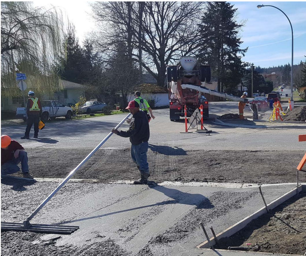
New concrete sidewalk and intersection crossing being installed at Seventh Street
