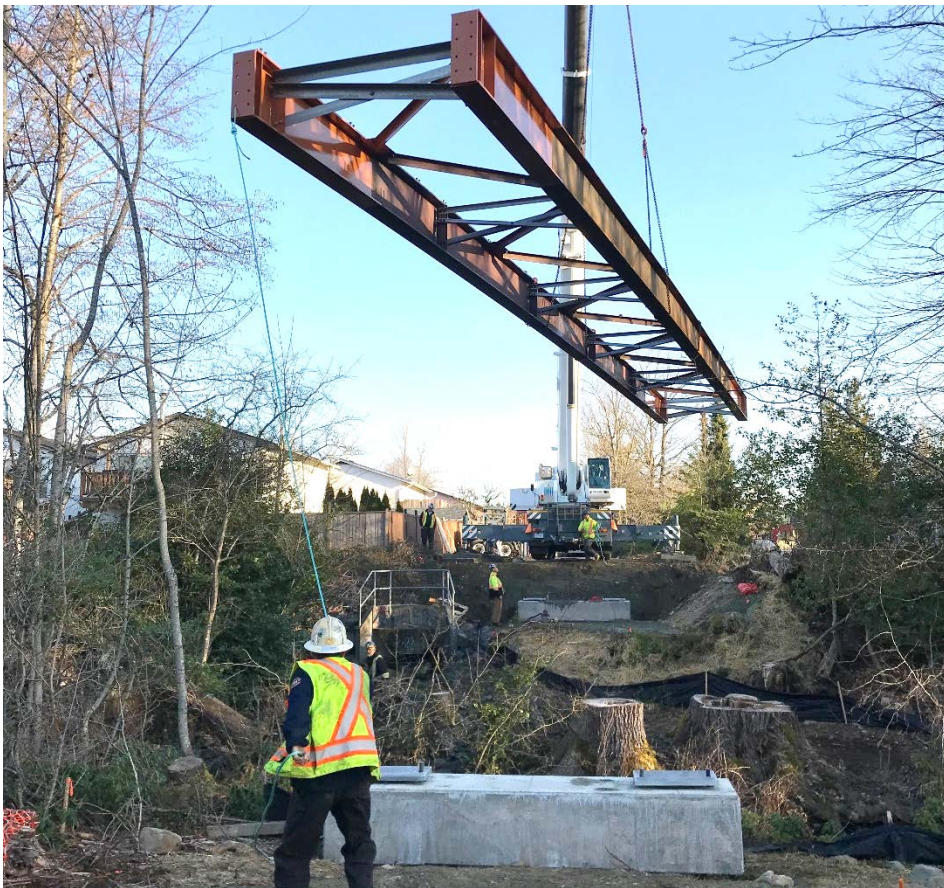
Steel bridge girders being lifted into place with crane
