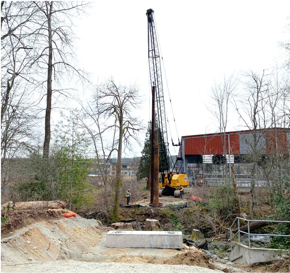
Pile driving for south bridge foundation
