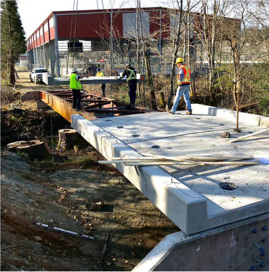
Precast concrete bridge panels being lifted into place with crane
