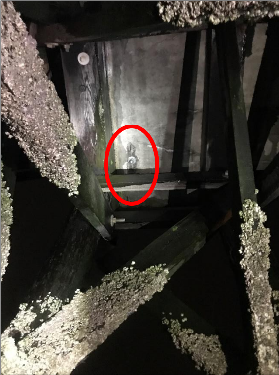
Photograph 3: Pre-cast hollow core deck panels, note: spalling at thru-bolt location
