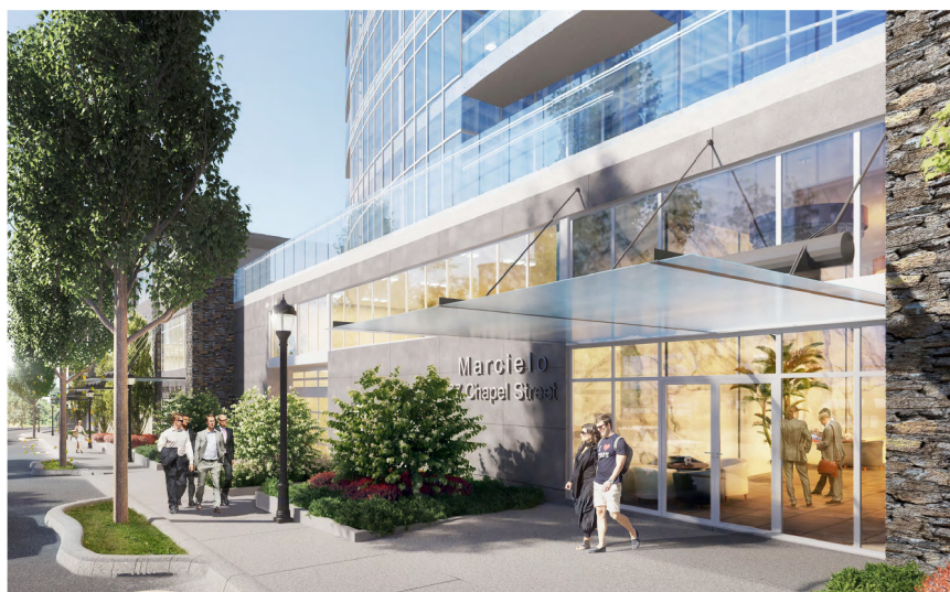
VIEW LOOKING SOUTH AT RESIDENTIAL ENTRANCE
