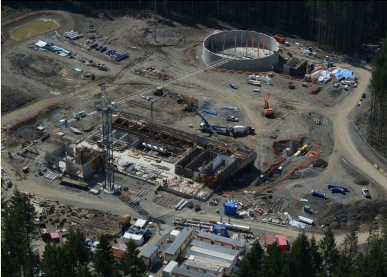
Construction of the new Water Treatment Plant building and clearwell – May 1, 2014
