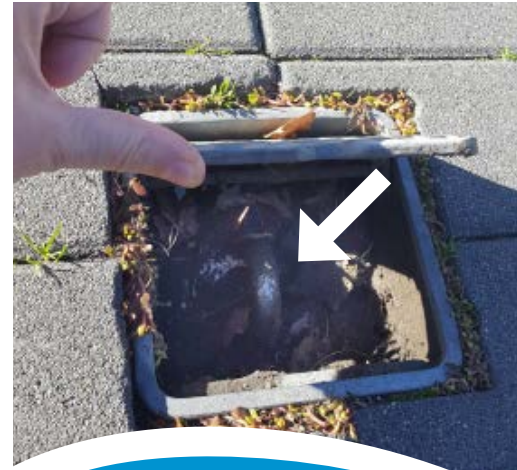
Tent tie-downs are located throughout Spirit Square to facilitate tent set-up and reduce the need for sandbags.
