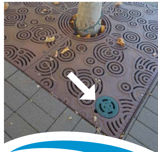
Power and potable water hook-ups are located throughout Spirit Square in removable tree grate discs to facilitate events set-up and reduce the need for stringing power cords across the plaza.
