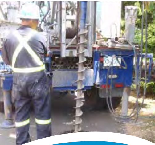
Truck-mounted auger drilling an archaeological test hole in Maffeo-Sutton Park during Spirit Square construction.
