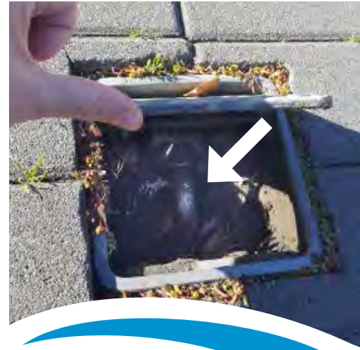
Tent tie-downs are located throughout Spirit Square to facilitate tent set-up and reduce the need for sandbags.
