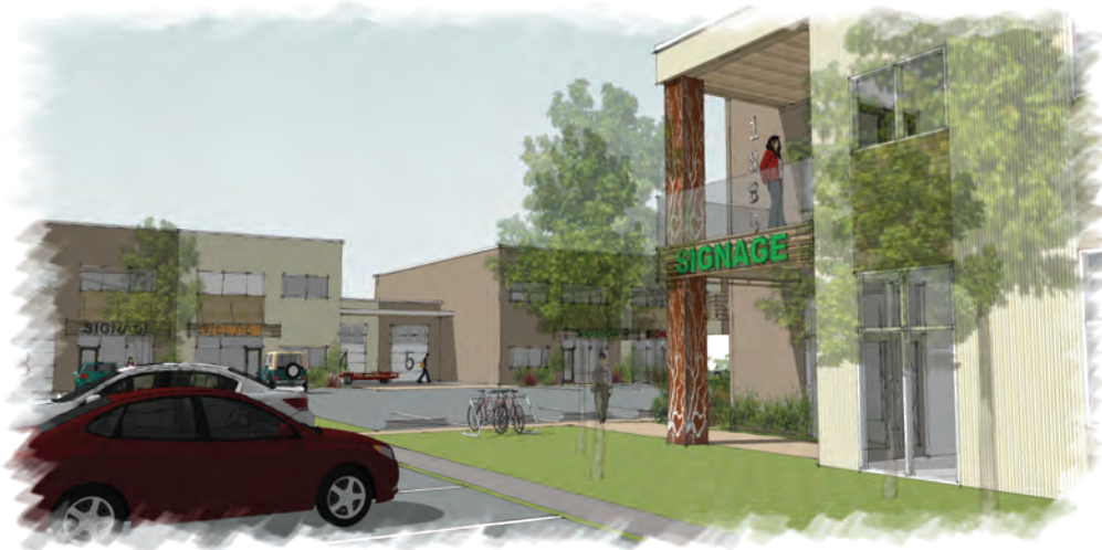
1 SW @ BUILDING A CORNER
