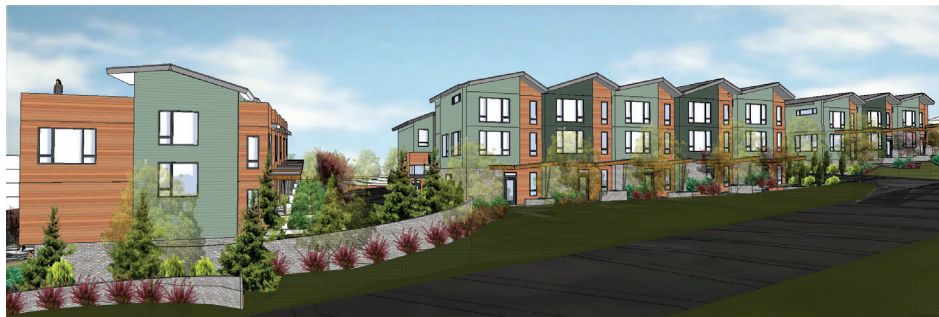
BUILDING 4 FROM STRONGTHARM ROAD
