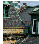
EXISTING HERITAGE- ROOF DORMER
