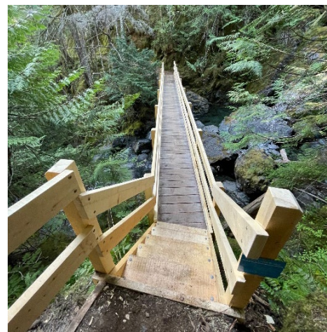
New handrail and steps on bridge
