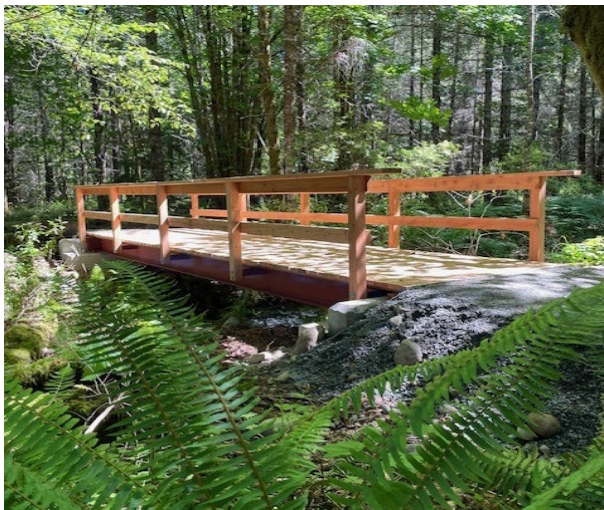
New bridge on Clay Banks Trail
