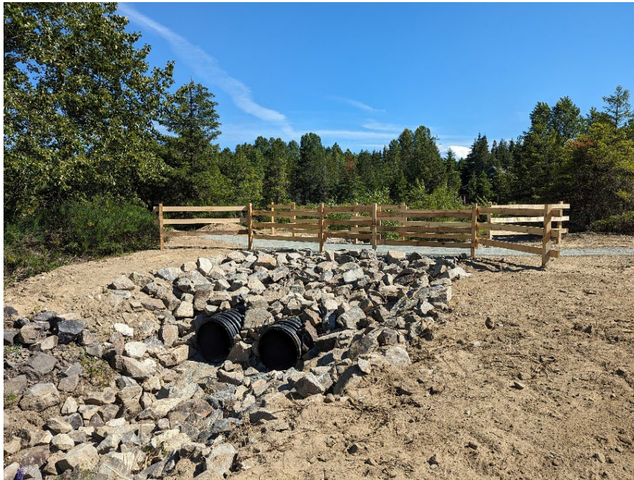
Photo of new culvert and trail crossing in Stormwater Community Park
