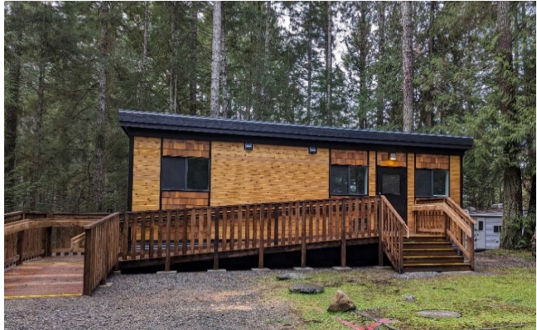
New prefabricated campground office building at Descanso Bay Regional Park.
