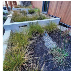
1. Terraced rain gardens along building.
