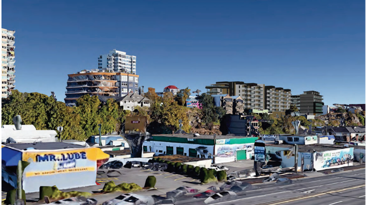
Looking South East along Terminal at Comox Road.
