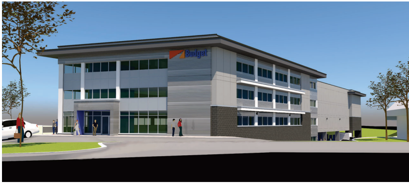
1 VIEW FROM SOUTH-WEST
