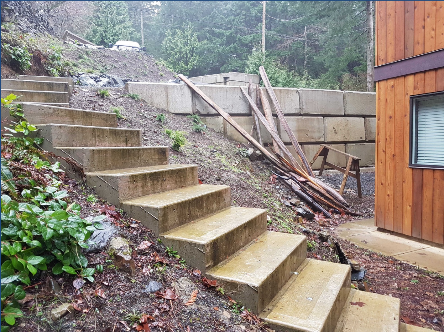
Access stairs from parking level. Handrail required on stair, and guard on retaining wall in background.
