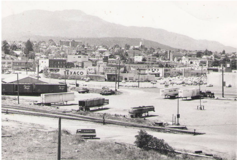
Photo 3: Photograph showing view of site in a westward direction in circa 1970.
