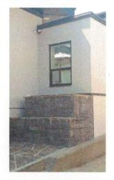
REVISION - DOOR & STAIRS REMOVED ADDED 3FT X 5FT WINDOW WITH 6FT X 4FT AND 1FT X 7FT TWO LEVEL STONE FACED PLANTER
