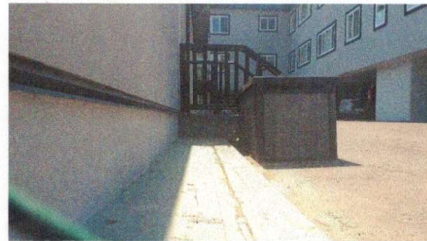
WESTERN ELEVATION PATIO ACCESS LANDING
