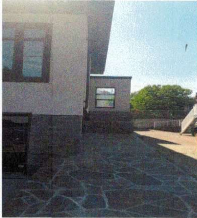
NORTH CORNER AT NEIGHBOURS DRIVEWAY
