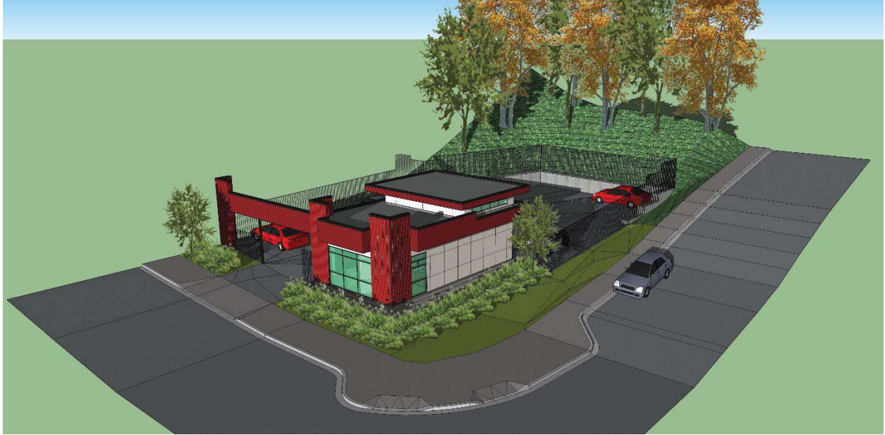
Aerial view of building at Fraser and Wentworth
