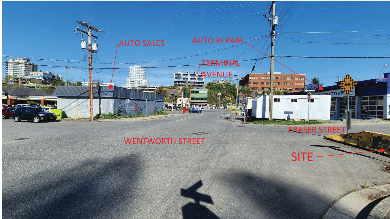
Fraser Street towards Terminal Avenue
