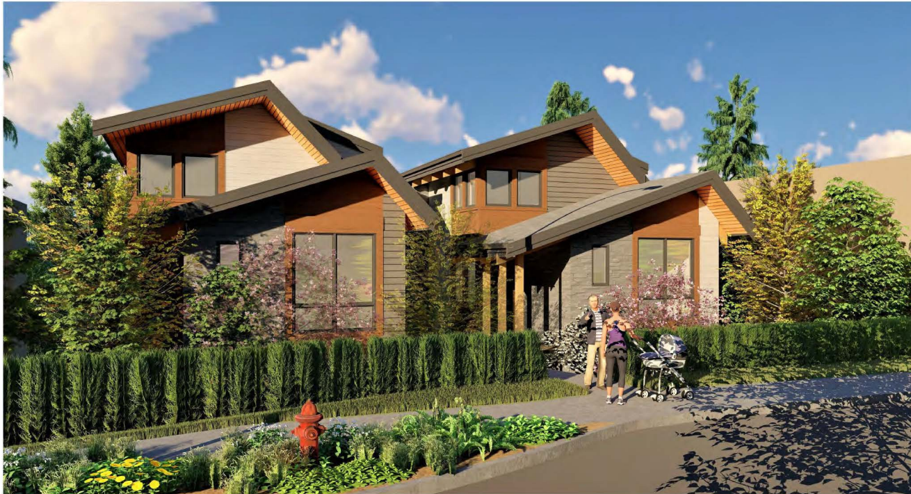
View from Milton Street
