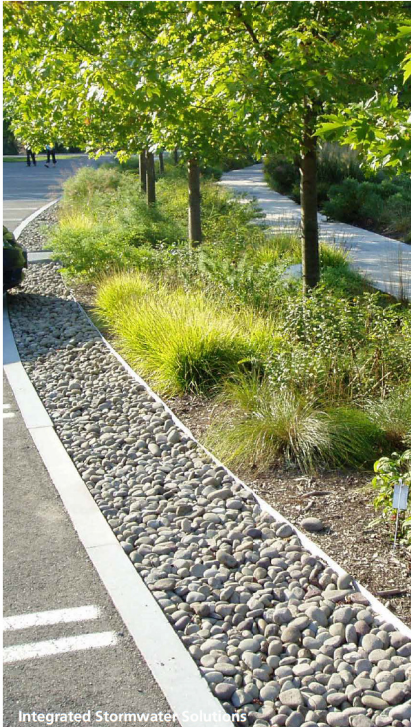
Integrated Stormwater Solutions
