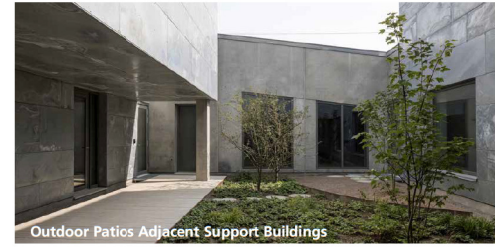
Outdoor Patios Adjacent Support Buildings
