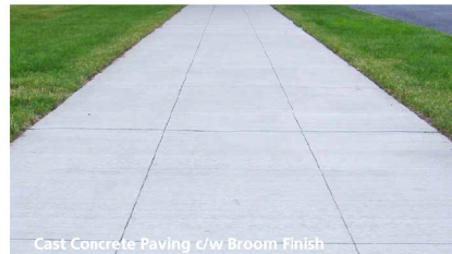
Cast Concrete Paving c/w Broom Finish
