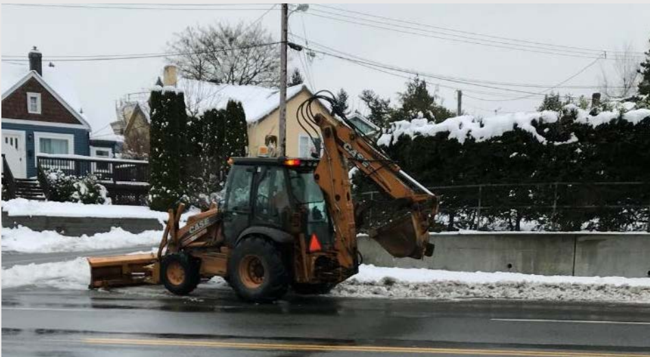
City plowing snow onto sidewalk & crosswalk on a bus route
