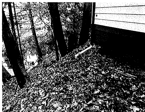
Photo 3 – Ground settlement at southeastern corner of #115
