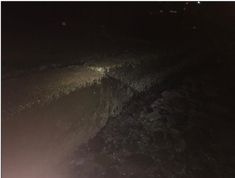
Photograph 6: Boat ramp, note: undermining of north side of ramp
