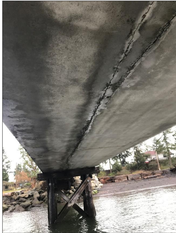
Photograph 2: Pre-cast hollow core deck panels, note: longitudinal crack penetrating the section, water seepage
