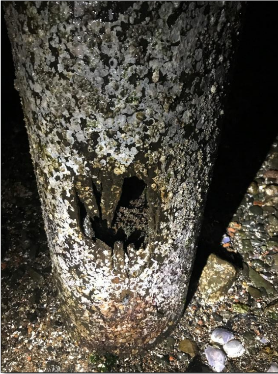
Photograph 5: Bearing Pile 4B, note: large hole with 80-90% CSL
