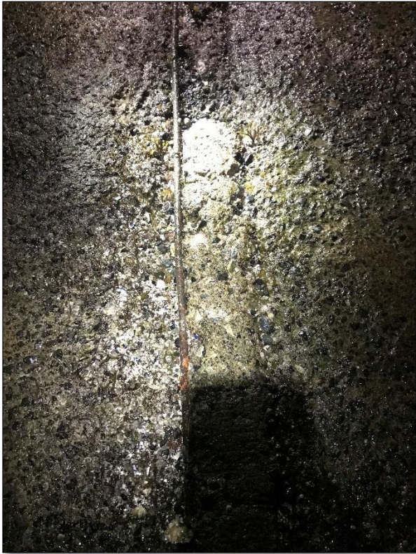
Photograph 7: Boat Ramp, note: spalling of the concrete panels with exposed reinforcing
