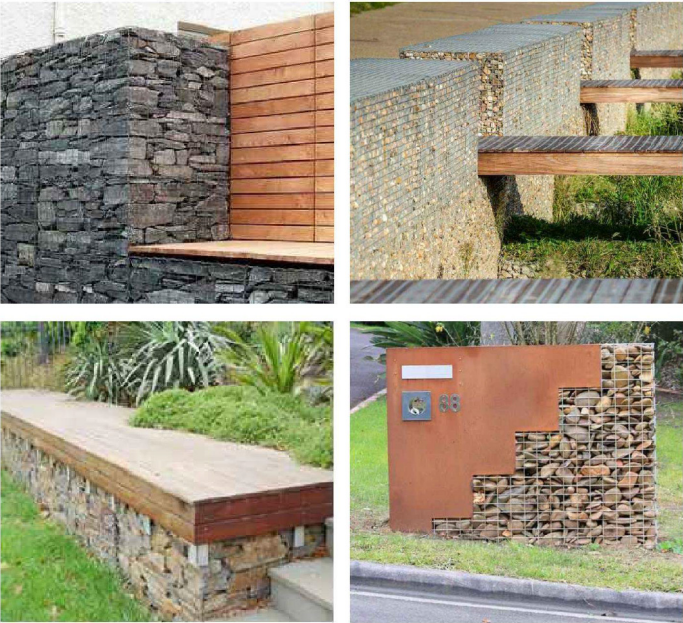
RECYCLE SITE MATERIALS - GABIONS
