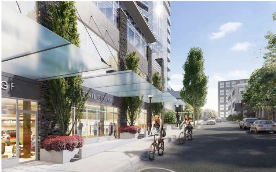
VIEW LOOKING NORTH ALONG CHAPEL STREET
