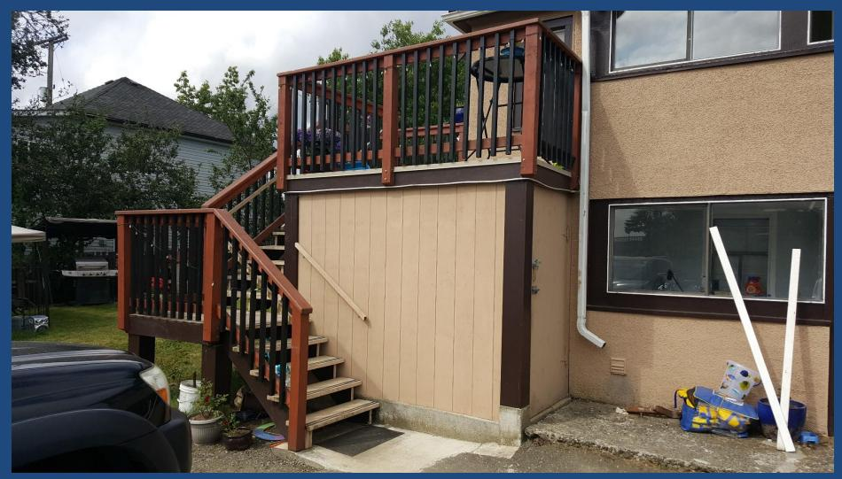
Handrail on stairs not long enough to go nosing to nosing. Closed-in room under stairs not part of approved permit.
