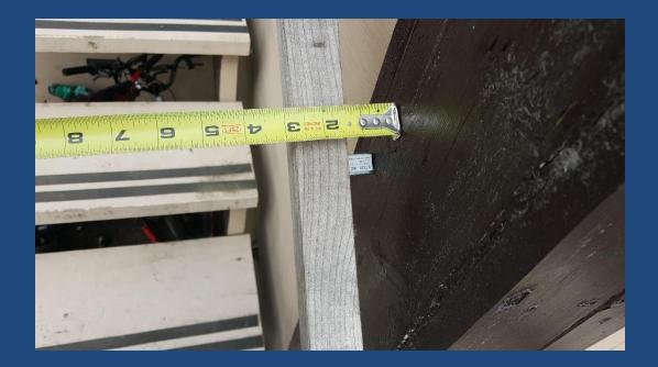
Upper handrail requires 2" clearance from wall to comply with building code.
