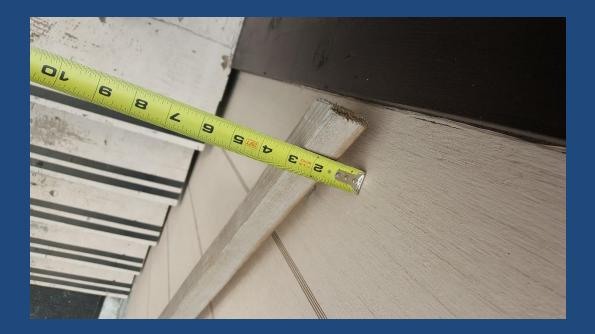
Lower handrail requires 2" clearance from wall to comply with building permit.
